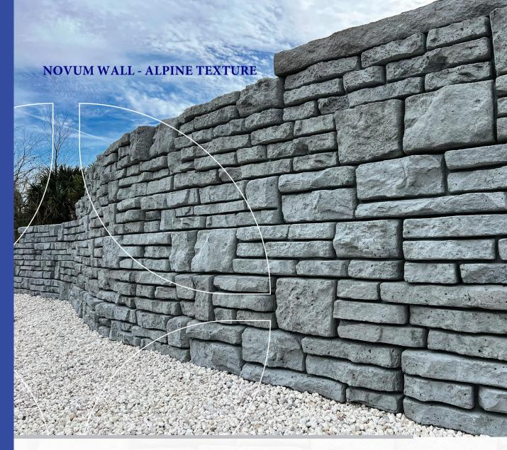
For gravity walls up to 6' tall, and the ability to use geo-grid for taller walls, Novum is the Wetcast, Machine-set block solution for your retaining wall needs. Fast installation keeps project costs low, while Superior Durability, and unique aesthetics with 9" block height give owners long-term satisfaction.
